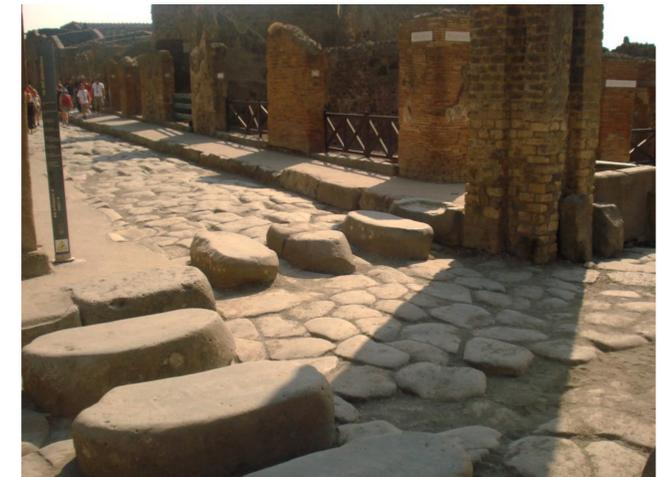
Figure 4. Road designed for exceedance flows with stepping stones
