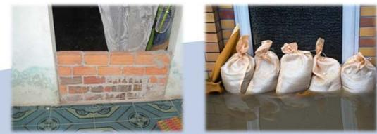
Fig. 1. Flood risk mitigation measures: Water barriers applied in Can Tho and Dresden
